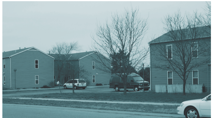
The Country Acres apartment complex before construction began earlier this year.
