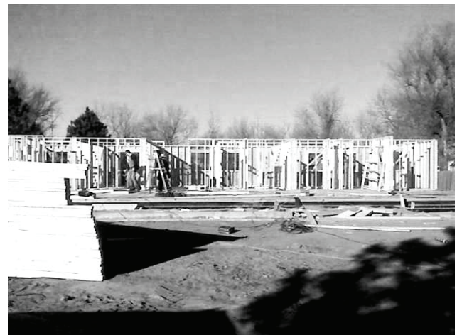
The 10th Street Project is making great progress. This housing development is focused on individuals with behavioral challenges.
